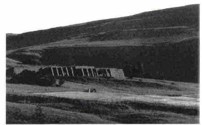
VIEW OF PRESS HOUSE, PHOTOGRAPHER BY MARCO ZANUSO SHORTLY AFTER COMPLETION OF WORK IN 1975
